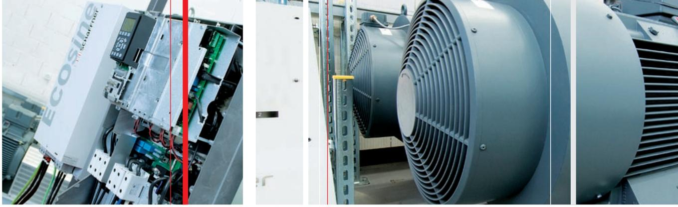
**Equipment longevity, reliable production uptime.** Because of their unique design, ECOSine™ filters add impedance to the supply, thus providing all the benefits of traditional Schaffner AC line reactors. In motor drive applications, for example, they eliminate nuisance tripping, and protect the rectifier and DC-link capacitors from mains transients. Longer equipment service life and reliable operation of mission-critical applications reduce cost of ownership and help safeguard profits.
